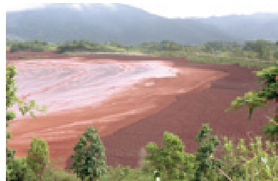
Figure 23.16 A lake of 'red mud', the waste from the pre-treatment of bauxite with sodium hydroxide
