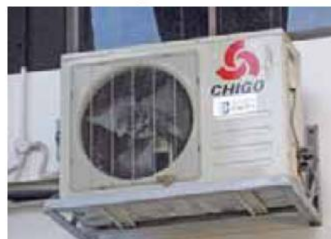
Figure 17.3 A domestic air conditioning unit
