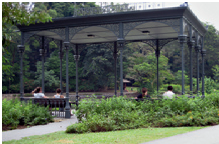
Figure 23.12 The cast iron gazebo in the Botanical Gardens, Singapore
