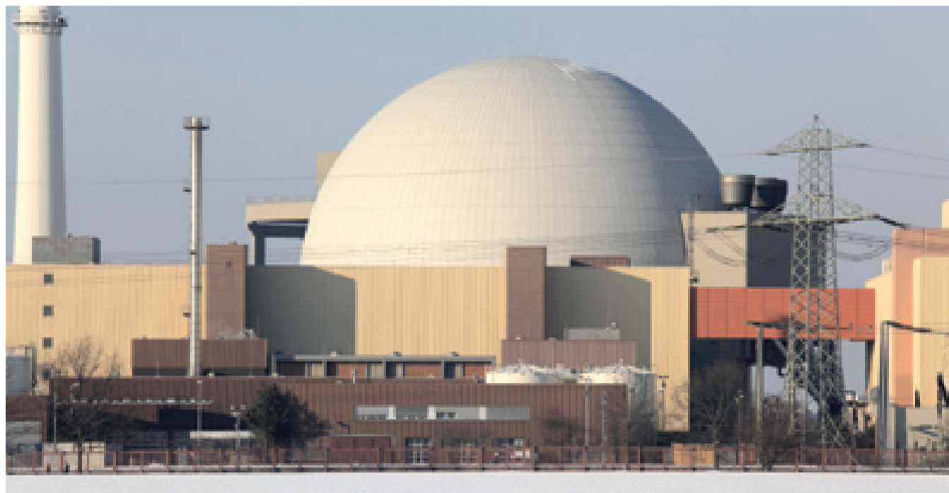
Figure 25.24 Nuclear reactor in a power station
